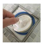
Pull the handle firmly upwards so the full NOOD water trap comes out of the drain.
