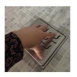
Place the square stainless steel grating back in place on top of the floor drain.
