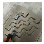
Remove the square stainless steel grating from the top of the drain. You can use a screwdriver or something similar to ease it out.
