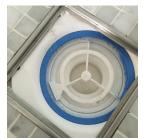
Once clean, place the NOOD water trap back into the floor drain and push it into position. Ensure the handle is clicked back into place.
