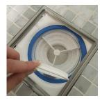
Locate the plastic circular handle from inside the floor drain and lift it upwards.
